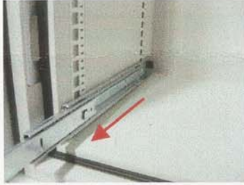
④ Pull out slide rail to remove from rail support.
